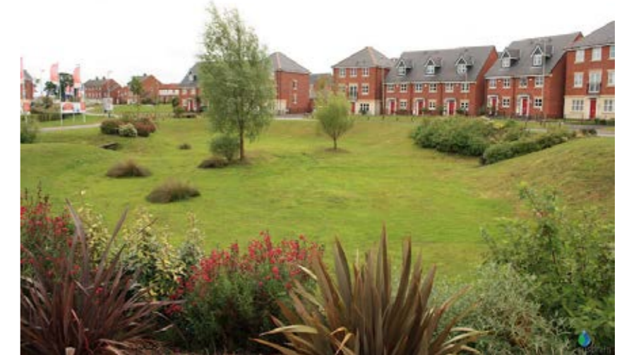
WELL-OVERLOOKED ATTENUATION BASIN
