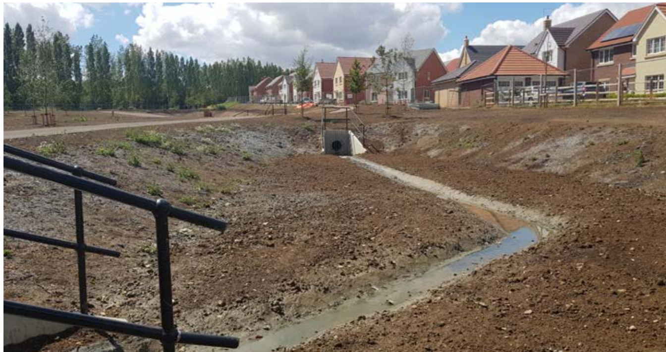
ATTENUATION BASIN (DAVENTRY) – AT CONSTRUCTION
