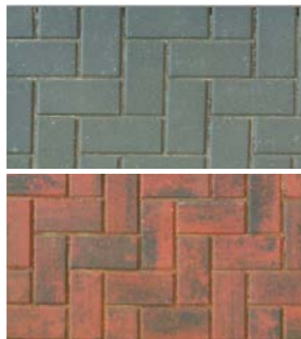
RAISED TABLES/PRIVATE DRIVES – BLOCK PAVING IN COLOUR GREY OR BRINDLE; VARIOUS PATTERNS OPTIONS
