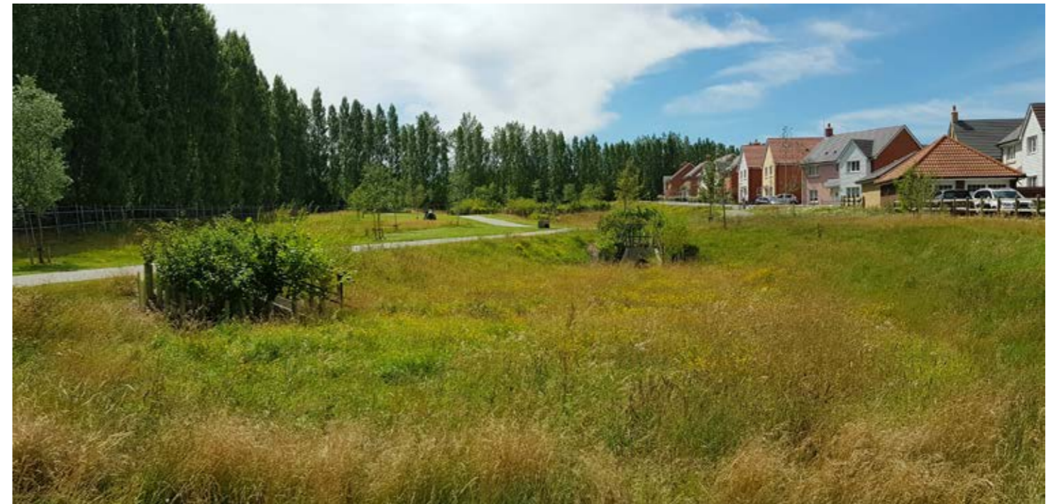
ATTENUATION BASIN (DAVENTRY) – AFTER ESTABLISHMENT OF LANDSCAPE
