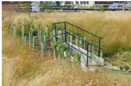
ILLUSTRATIVE EXAMPLE YOUNG NATIVE SHRUB PLANTING BEHIND HEADWALLS WHICH TO DISCOURAGE ACCESS
