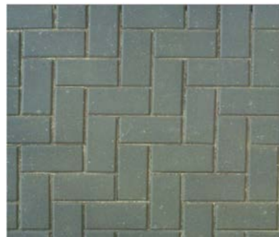
SHARED SURFACES – BLOCK PAVING – COLOUR: GREY
