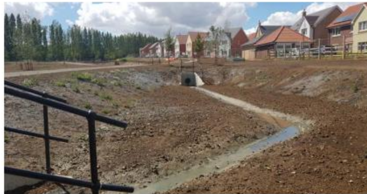
ATTENUATION BASIN (DAVENTRY) - AT CONSTRUCTION
