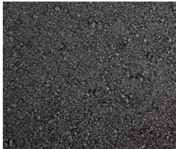
MINOR ACCESS ROAD – STANDARD TARMAC
