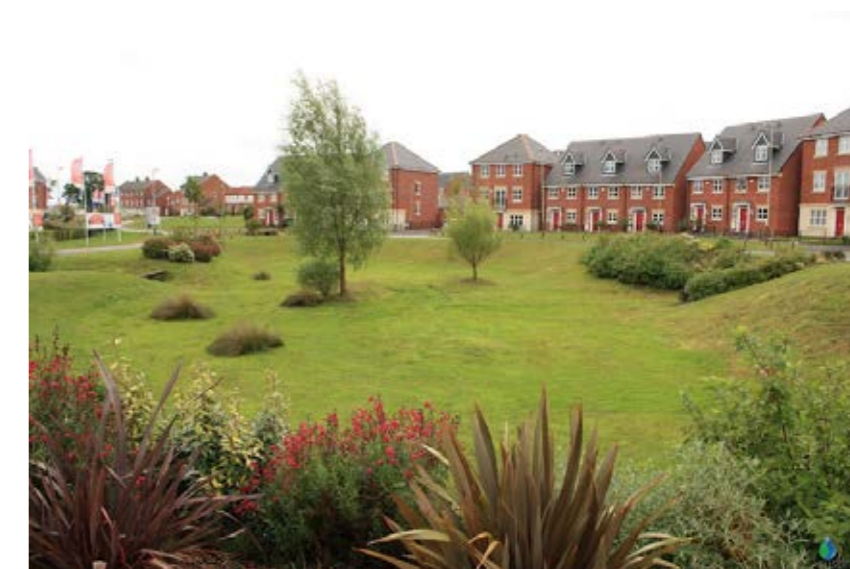
WELL-OVERLOOKED ATTENUATION BASIN
